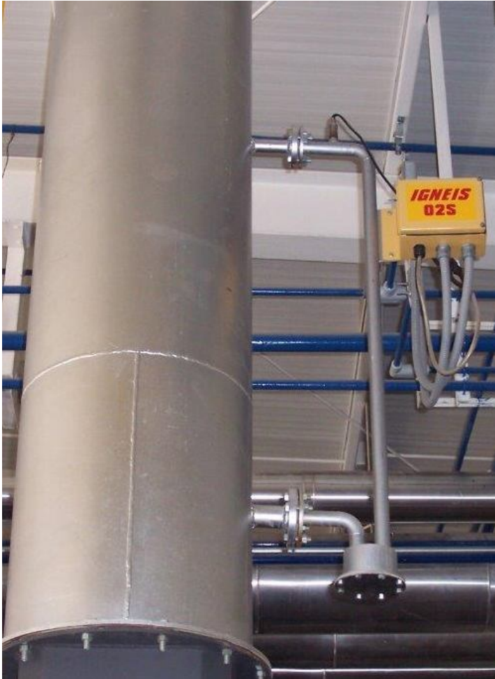
Stack mounted with measuring tube
